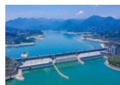
Power Station Reservoir
