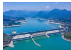
Power Station Reservoir
